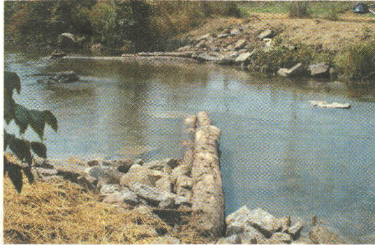
At the Sheep Farm Project, multi-log vane deflectors and instream habitat boulders.
