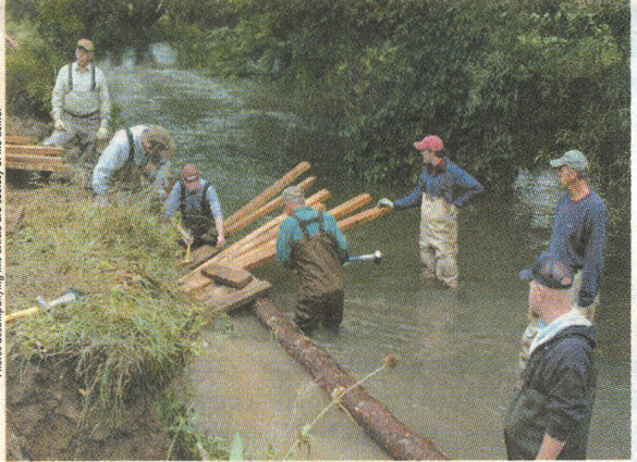
The crew constructing a mudsill on Spring Creek
